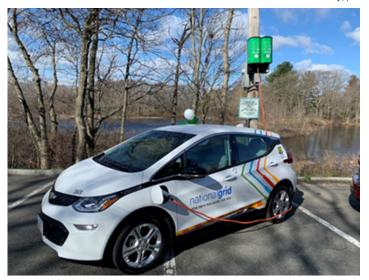
Setups like this Melrose, Massachusetts, pole-mounted charging station can help in situations where residential chargers are not possible. Photo: Voltrek LLC
